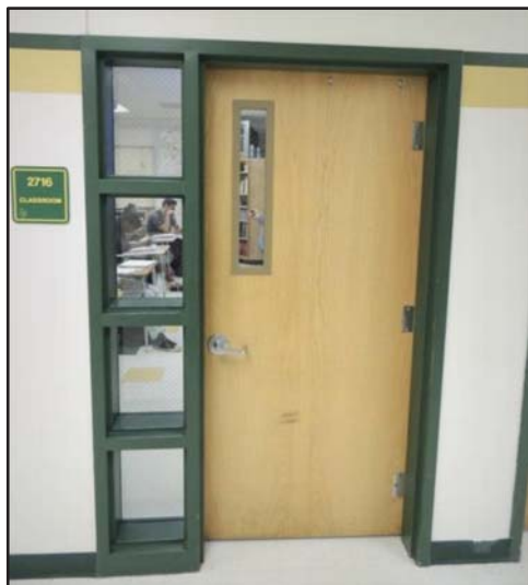
Figure 22: Example of non-ballistic resistant glass near and in door, creating vulnerability to assailants.
