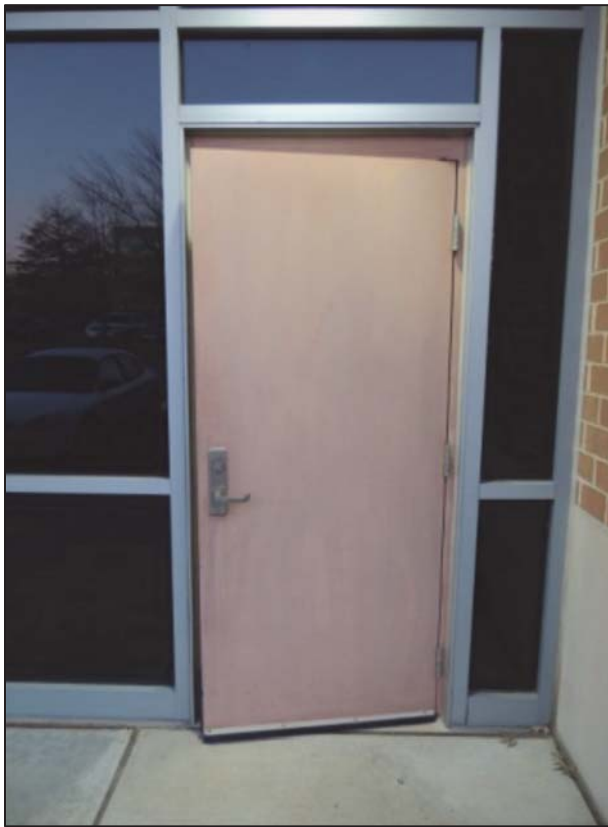
Figure 155: Unprotected hinges.
