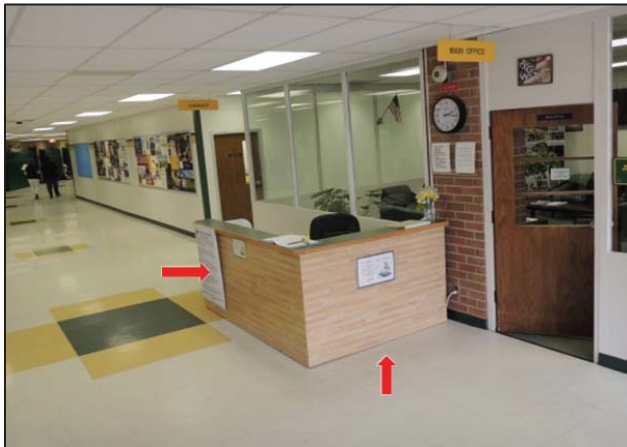
Figure 12: Red arrows indicate ballistic steel plating.
