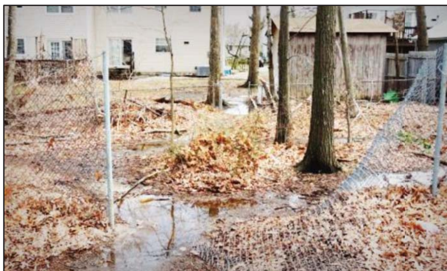
Figure 2: Inadequate perimeter fence.
